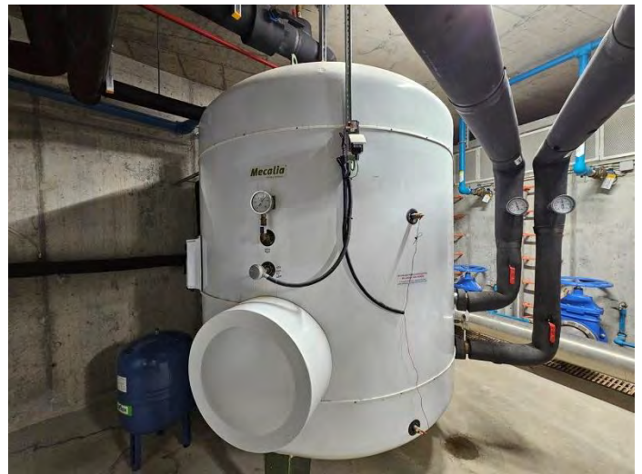
Figure 8: DHW accumulator
