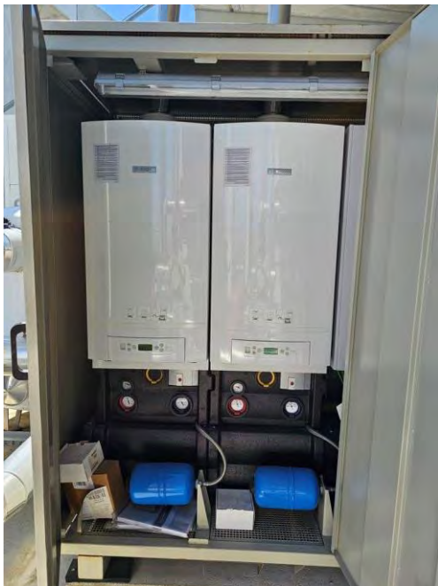
Figure 7: Residential condensing boilers
